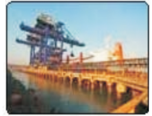
JSW Jaigarh Port Ratnagiri
