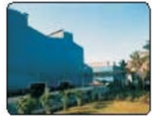
JSW Steel Tarapur
